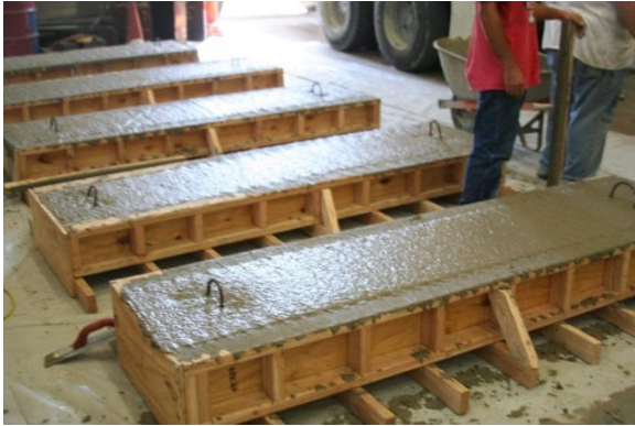
Figure 121. Five of 12 Completed SFRC Slab Strips
