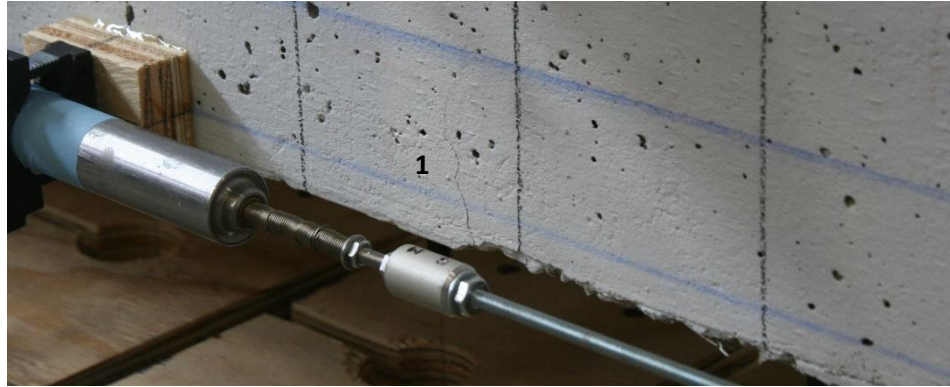
Figure 273. S7520NOS00 Damaged Corner
