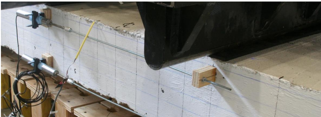
Figure 235. S7505BTM24 Damaged Corner
