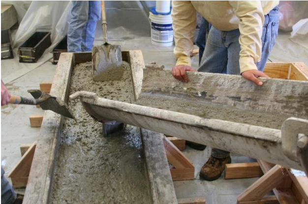
Figure 120. Placing Concrete Directly into Forms
