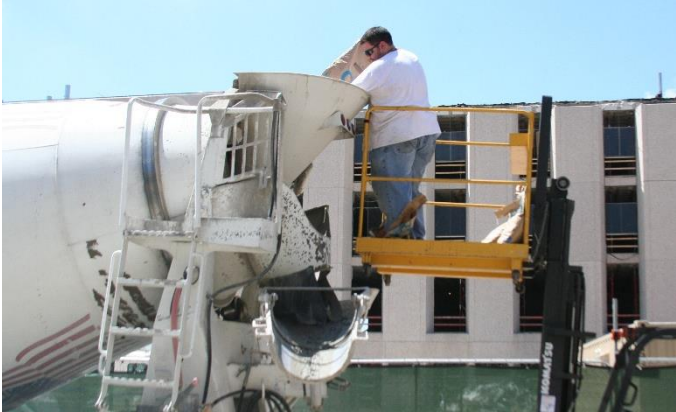
Figure 118. Adding Steel Fibers to Concrete Truck
