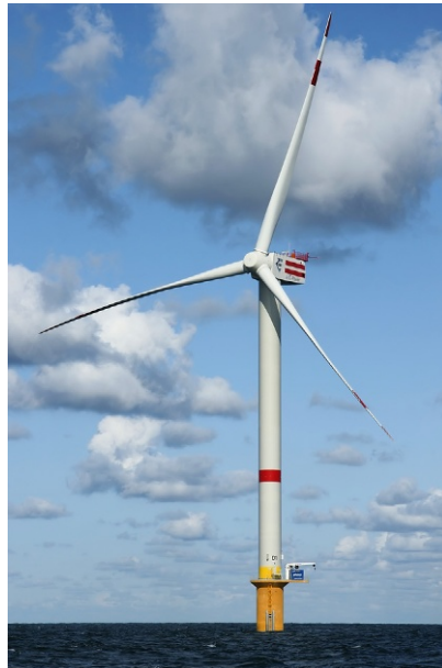
Fig. 3.3 A 157 m high wind turbine at the North Sea [8].
