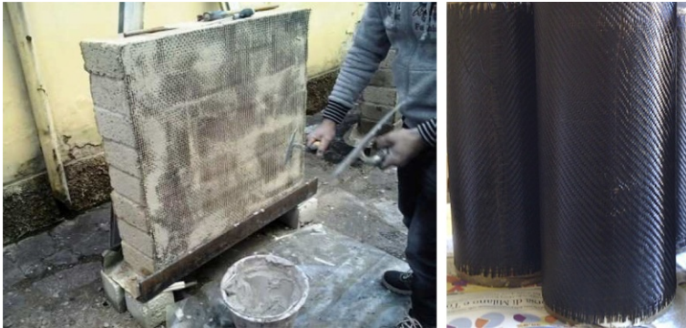
Fig. 8.10 External strengthening of the structures with basalt-based materials.
