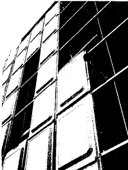
Figure 8.9 GRC precast cladding panels: (a) As cast; (b) assembled in a structure. Photographs courtesy of Pilkington Brothers PLC, UK.
