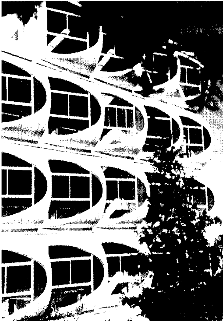
Figure 1.2 Industrial engineering building, Technion, Haifa, Israel, made with complex shaped panels of glass fibre reinforced cement (Architect Y. Rechter).
