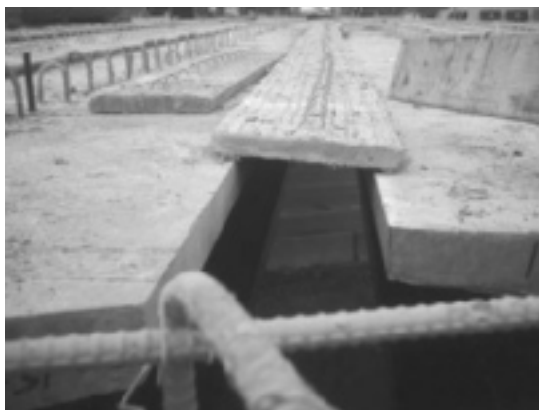
Figure 14.19 Stay in place formwork panels from fibre reinforced concrete, Photo by Finn Hubbard Wisconsin Department of Transportation.
