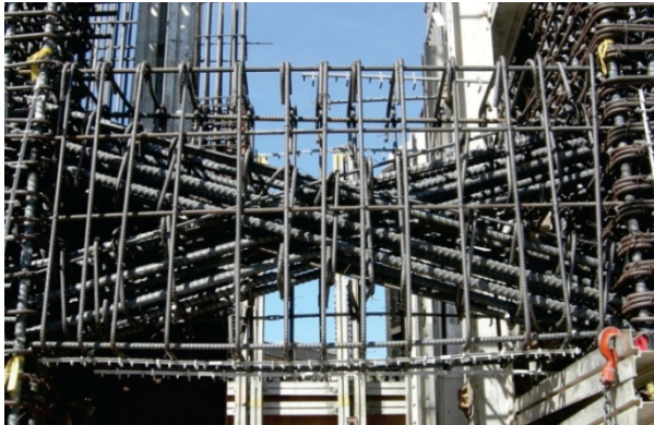
Fig. 1. Reinforcement detailing in diagonally reinforced coupling beam
