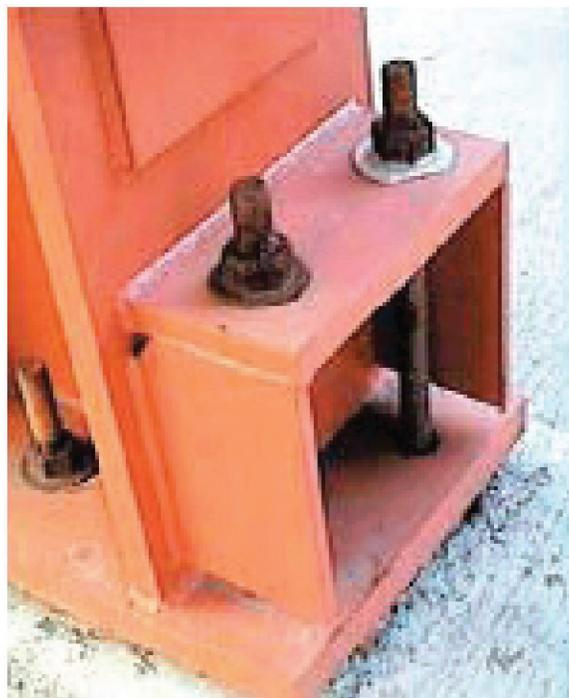
*Fig. A-2. Column moment base using an anchor rod chair.*
