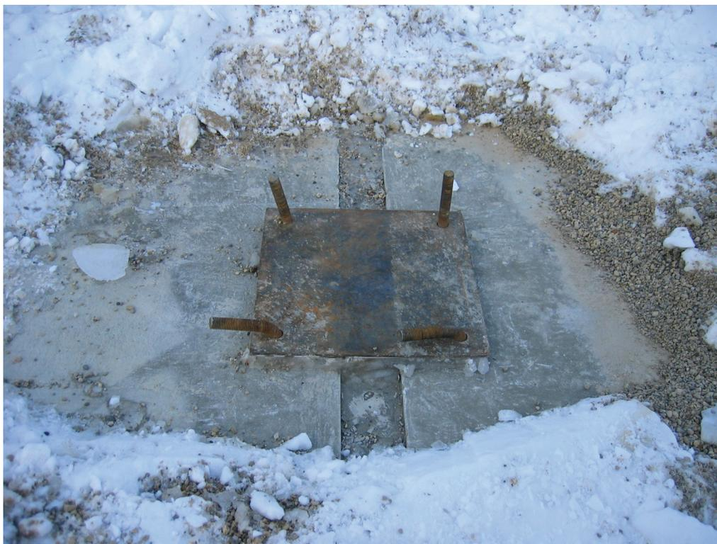
*Fig. 4-17. Anchor rods run over by a crane.*
