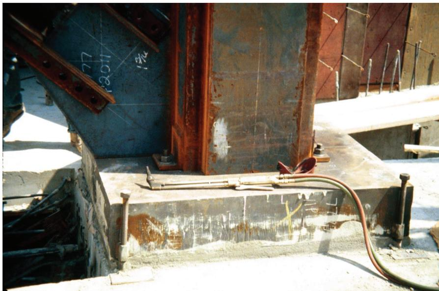
Fig. 4-16. Base plate with adjusting screws.
