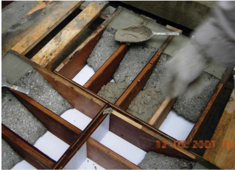
Figure 6-38 Casting of prisms for slant shear measurement
