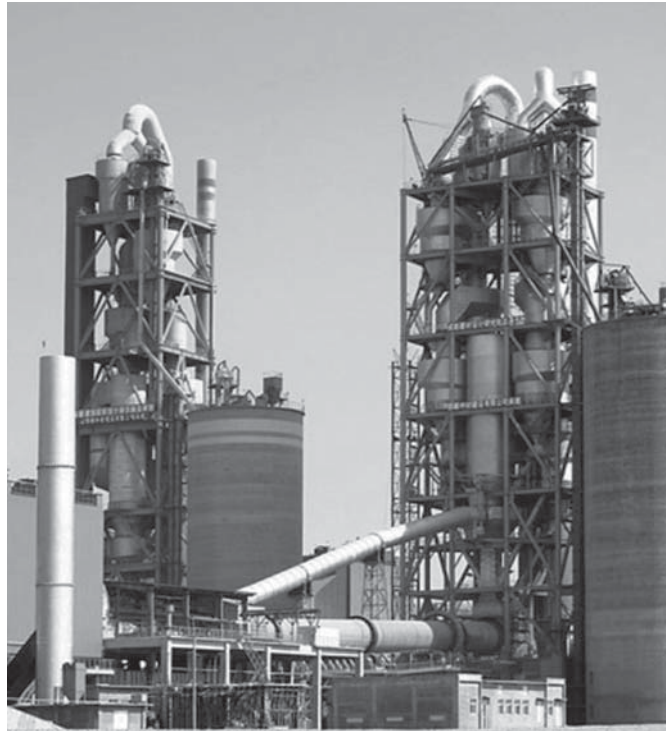
Figure 2-10 A production line of 10,000 metric tons per day (Hai Luo Cement Company, China)
