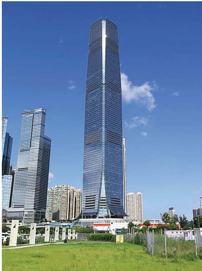
Figure 1-6 International Commerce Centre, Hong Kong. (Source: Wing1990hk / Wikimedia Commons / CC BY-SA 3.0)
