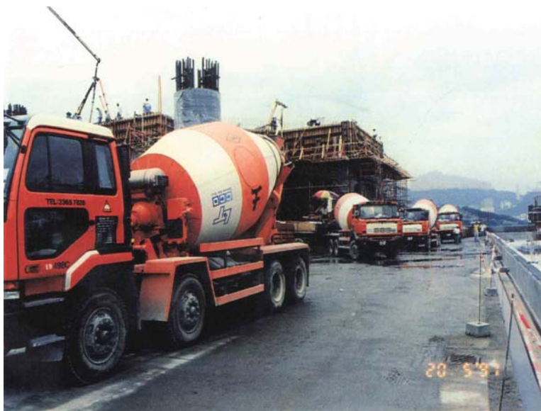
Figure 3-22 Delivery of concrete by truck
