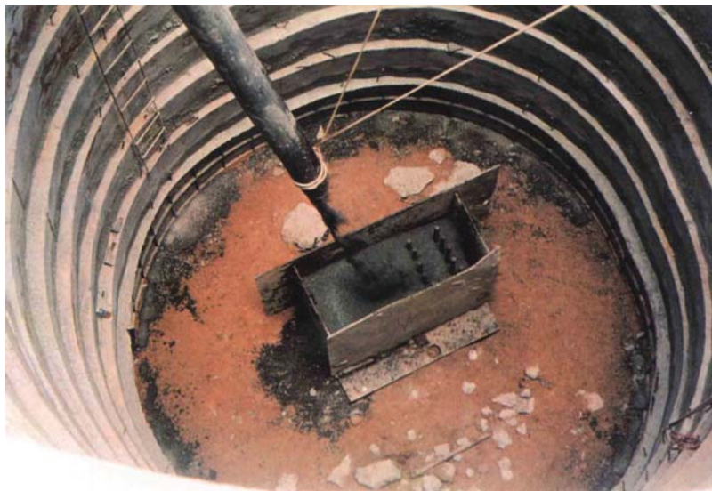
Figure 3-30 Drop chute-guided concrete fall
