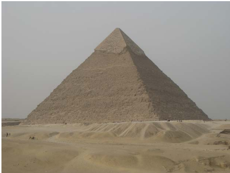
Figure 1-1 Pyramid built with gypsum mortar, Giza, Egypt
