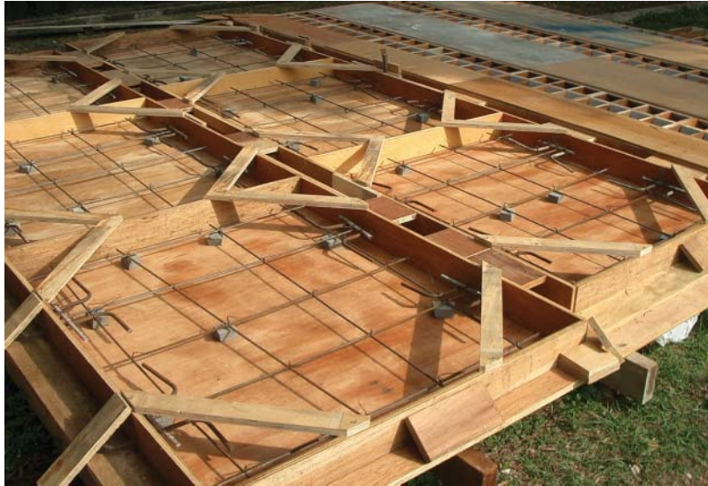
Figure 1-14 Formwork for concrete casting
