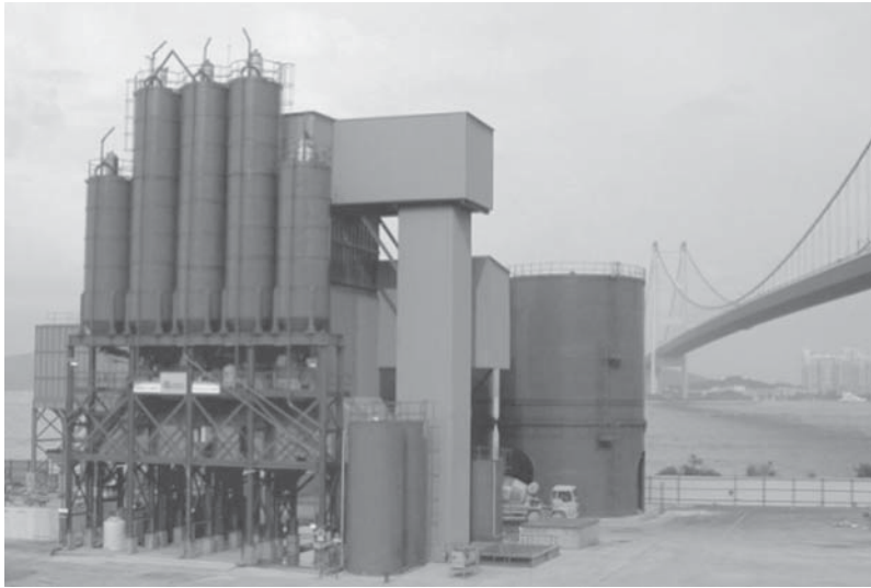
Figure 3-20 Ready-mix concrete plant
