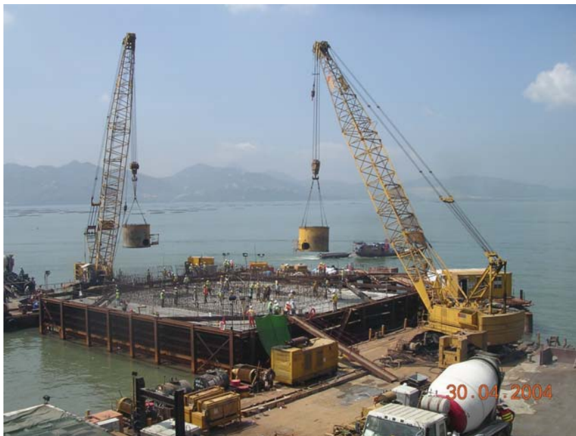
Figure 3-27 Unloading concrete (Photo provided by Ove Arup, HK)
