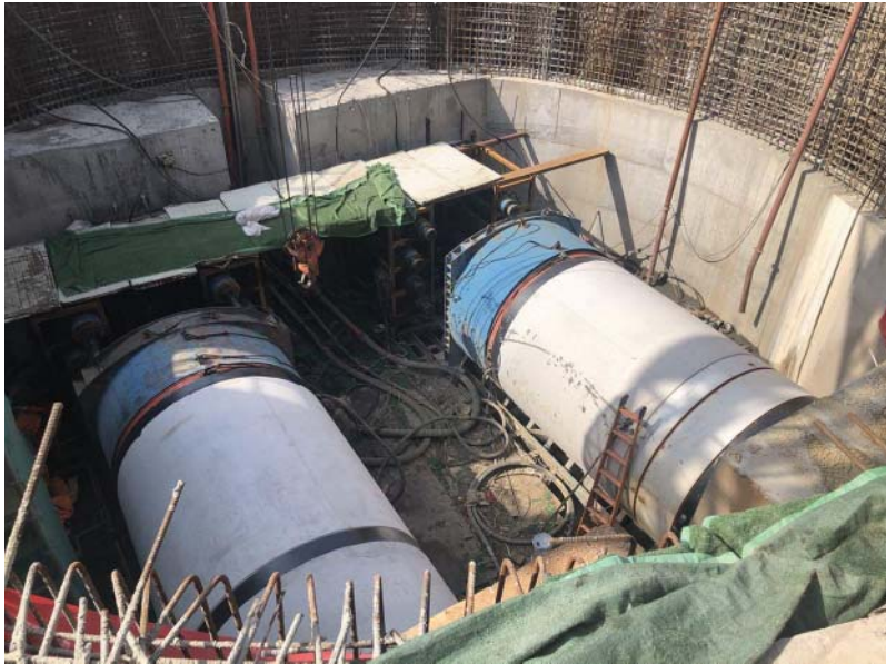
Figure 1-11 Pipeline under construction (Photo provided by Zhulin Zhang)
