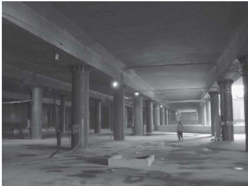
Figure 6-53 Application of CFST as short axially load column in Tianjin Station, China (Photo provided by Linhai Han)
